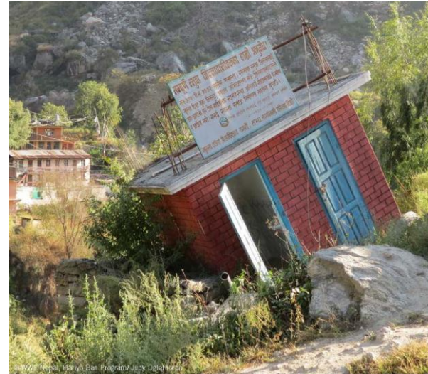
Public toilet damaged by the earthquake in Rasuwa
