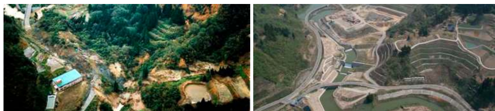
Chuetsu Earthquake; 2004, Niigata Pref., Japan (Left: Just after occurrence, Right: Countermeasures completed)
