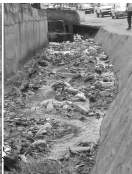
Figure 14: Clogged gutter in Accra
