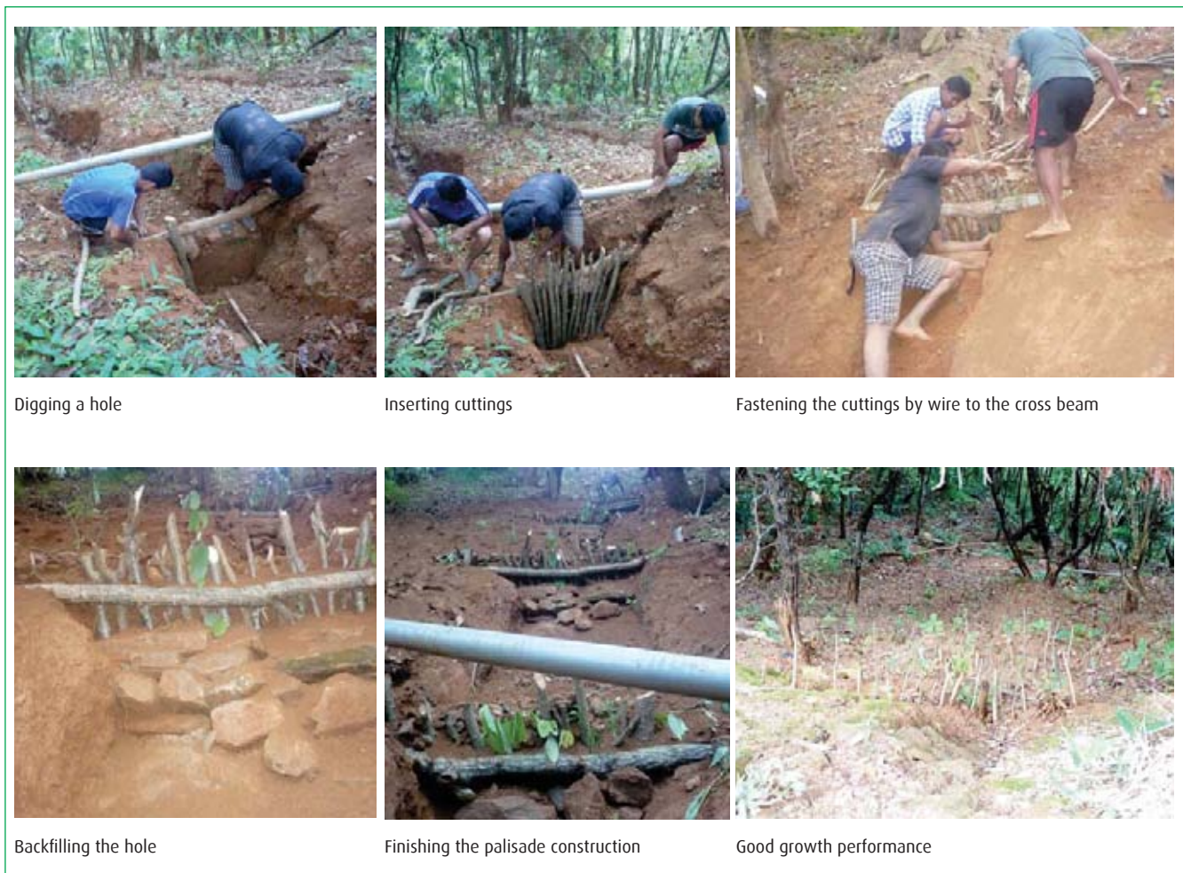
Figure 6: Construction steps for palisades in series to protect a long, narrow gully (Dhodre, Gorkha).
