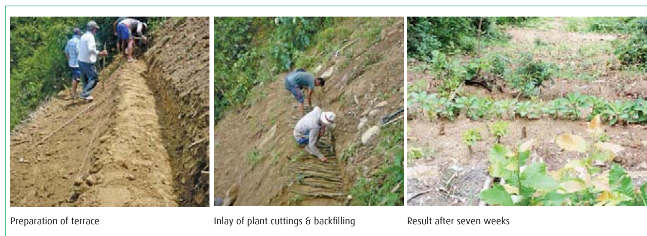
Figure 3: Construction steps of brush layering (Dhodre, Gorkha)
