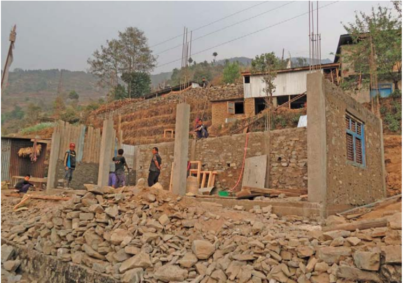
Reconstructing a building in Rasuwa district after the 2015 earthquake with a mixture of old and new building materials. © WWF Nepal, Hariyo Ban Program/Judy Oglethorpe
