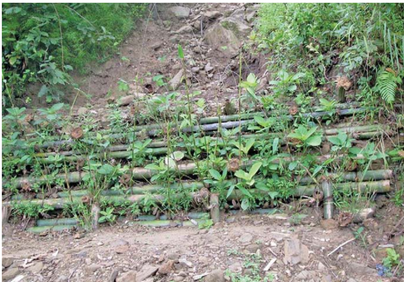
Bamboo crib wall after 10 weeks (Dhodre, Gorkha) © WWF, Hariyo Ban Program/Madhuban Lal Maskay
