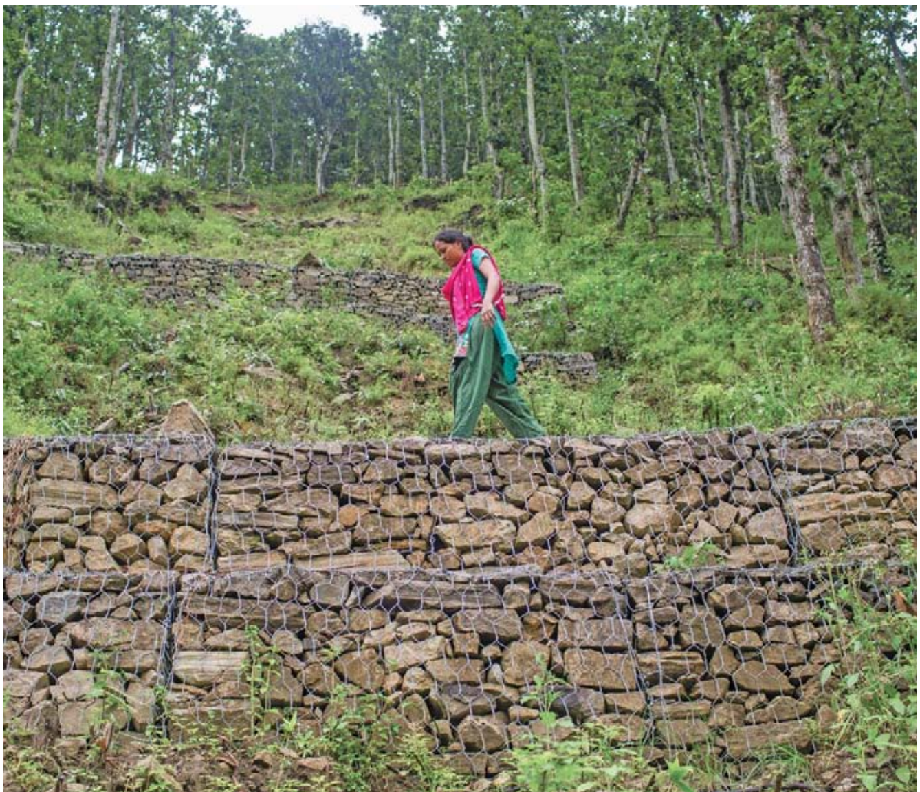
Kamala Ghale in Pairobesi participated in restoring this landslide which was threatening her village; a combination of gabions and soil bioengineering was used to stabilize the slope.
