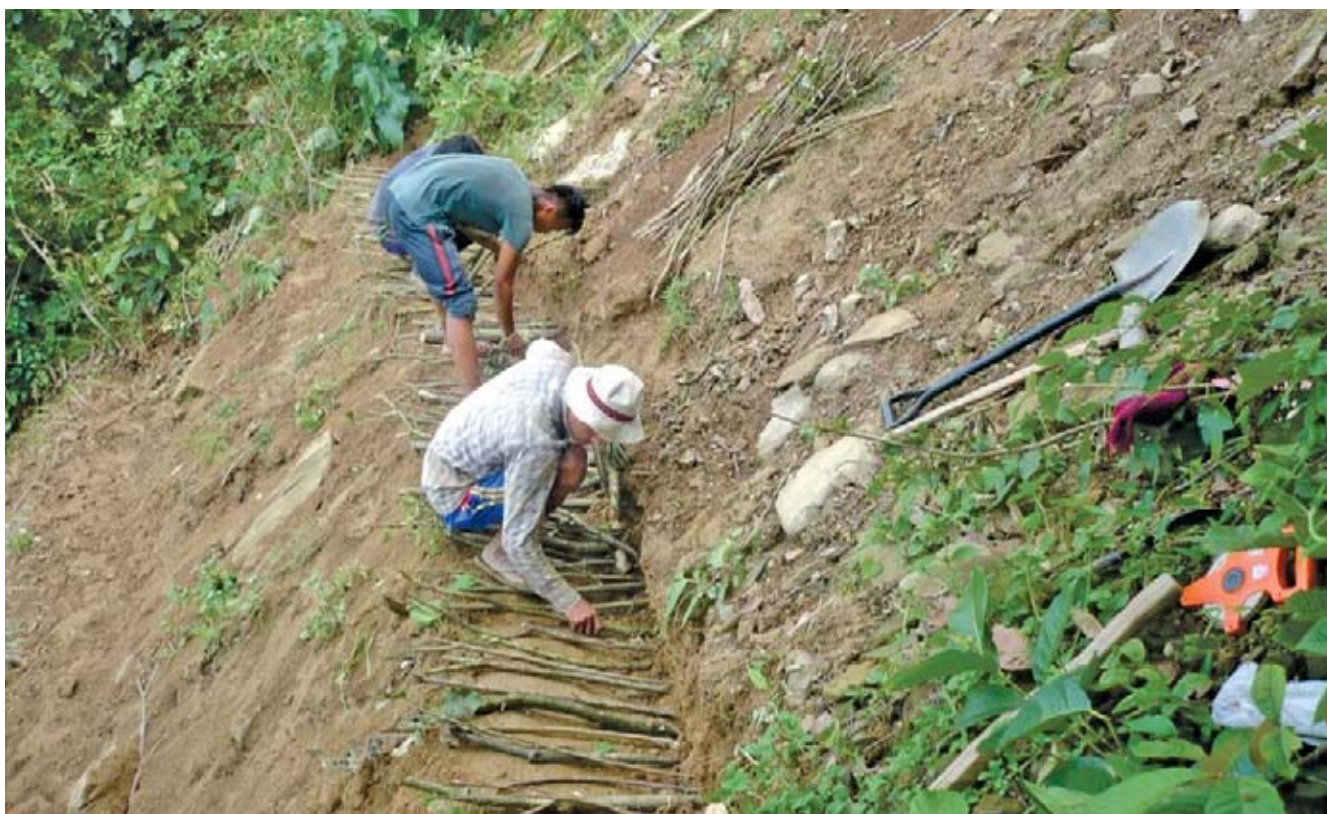
Constructing brush layer (Dhodre, Gorkha) © WWF, Hariyo Ban Program/Madhuban Lal Maskay
