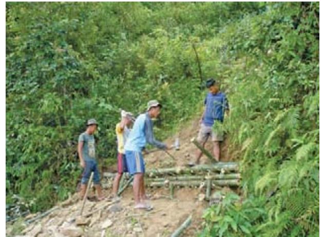
Live cuttings inserted between first and second layer stretchers
