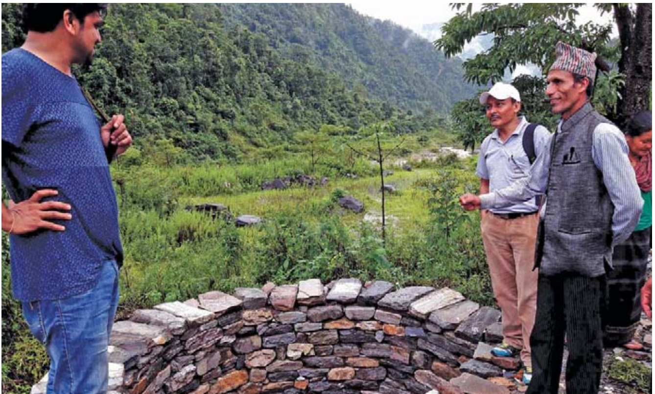
Newly constructed garbage pit for waste management in Jeevan Jyoti Lower Secondary School, Simjung 9, Gorkha district, part of a program to promote green recovery and reconstruction in schools after the 2105 earthquake. The garbage is collected in the pit and burned periodically. © CARE Nepal, Hariyo Ban Program/Binita Khanal
