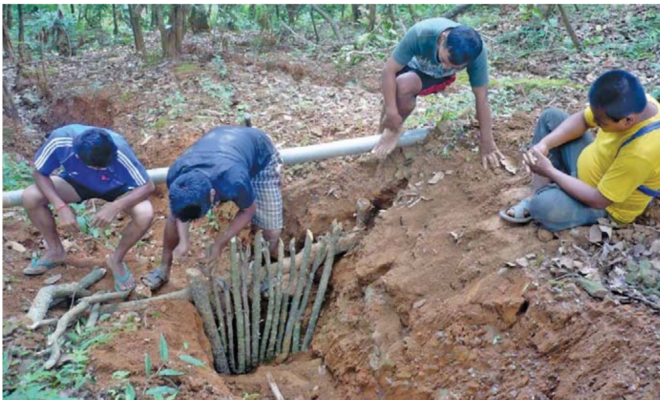
Constructing Palisades in series to protect a long, narrow gully © WWF, Hariyo Ban Program/Madhuban Lal Maskay
